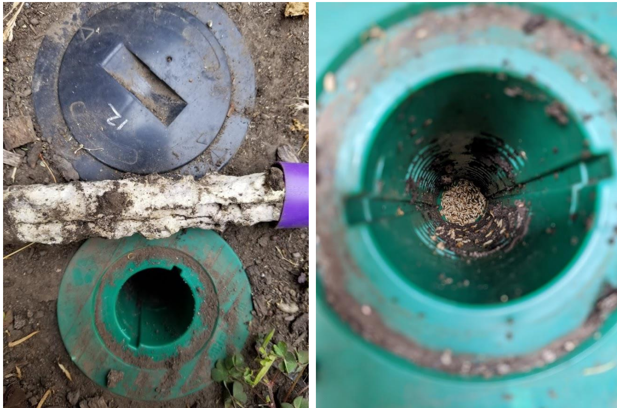
Figure 1. Sentricon Always Active bait tube damaged by termites (left) and associated bait station containing termites (right) approximately six months after installation at Berkeley site.
