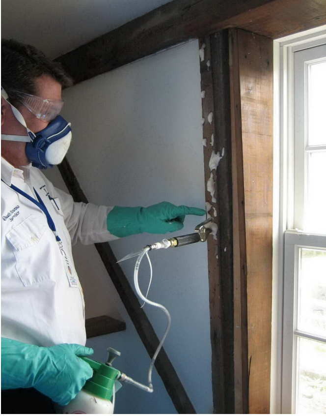
Figure 4. Example of injecting Optigard into infested board; location Petaluma, CA. Included in image is M. Red, Clark Pest Control.
